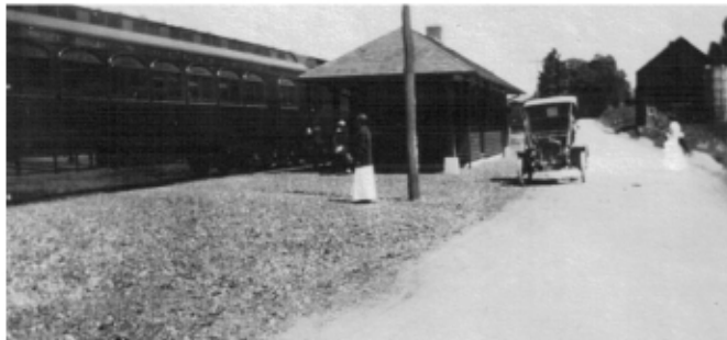
Kelly Corners U&D passenger depot, looking north on Rte 30
