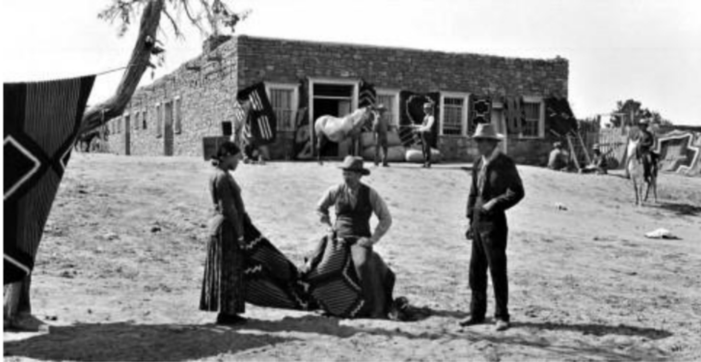
Hubbell buying a rug on the north wall of the post, probably from the Navajo weaver, circa 1897 (NPS, Hubbell Trading Post NHS; HUTR 2165)
